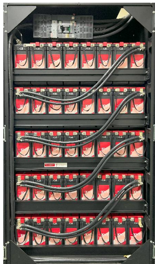
XHT9000FT Battery Cabinet 480Vdc
