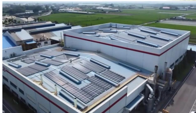
Tainan Plant with PV Array - Installed Dec 2022. Expected to remove 365MT of CO 2 emissions annually (equivalent to removing 4,101km of car emissions daily)
